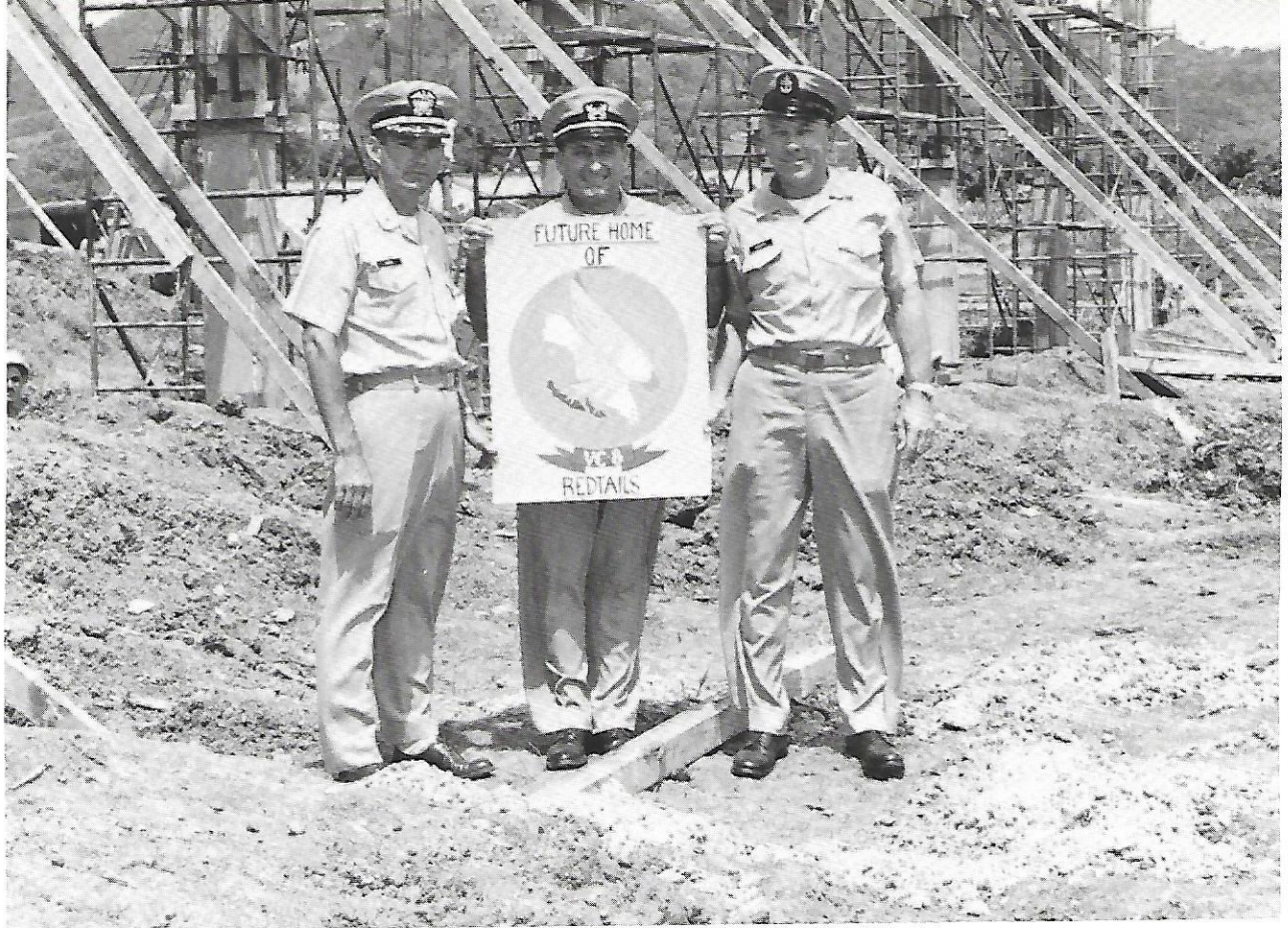
Skipper, WO-2 Spata and Chief Roberts inspect construction of new hangar.
