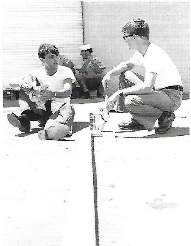
J. T. Sheerin and W.R. Prayner paint yellow lines on new parking lot.
